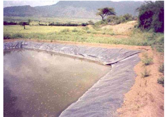
Cheaper than concrete: Plastic lined pond Alamata
