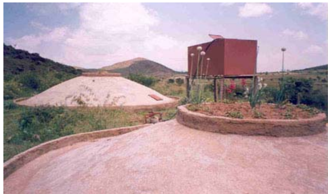
Onions growing on top of dome shaped water-harvesting tank: Trial site in Adama, East Shewa (photo H. Rami, UN-OCHA, Sept 2003)
