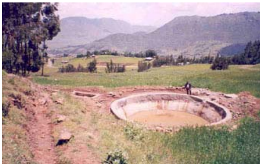
Leaking from outside in: Hemispherical tank built on a slope in Dessie Zuria with groundwater seeping through the walls into the tank (photo H. Rami, UN-OCHA, Oct.
