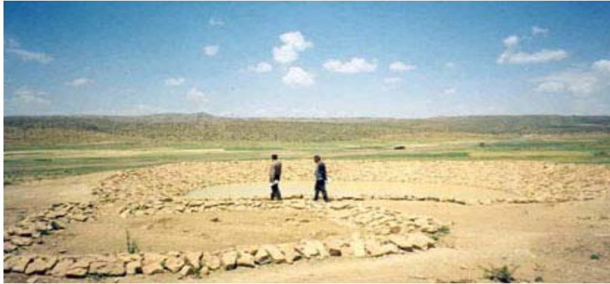
Rapid siltation: Full silt trap due to lack of watershed treatment, Geteb Dawru watershed (photo H.Rämi, UN-OCHA, Oct 03)
