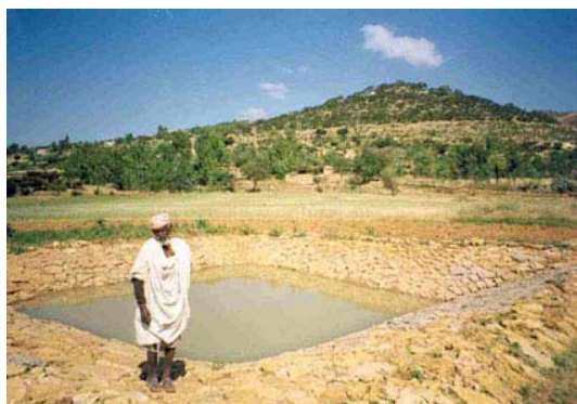
Supplementary irrigation during dry spells: Farmer with his plastic lined pond, covered by stones in Wukro woreda (photo H. Rami, UN-OCHA, Oct. 2003)
