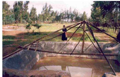
Never filled up: Tank built for poor women's cooperative in an area without water catchment (photo Rami, UN-OCHA, Oct. 2003).
