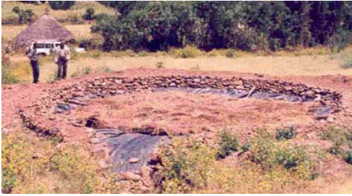
Lack of materials: Plastic lining instead of concrete in hemispherical excavation (photo H. Rami, Oct 03)
