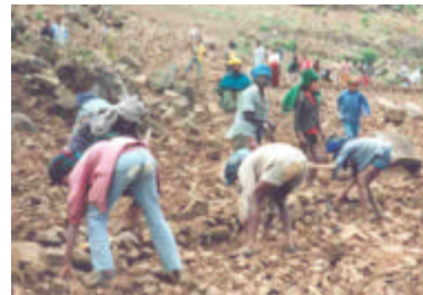
EGS- work on stone-bunds
