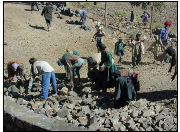
Cash-for-Relief rural road construction in Northern Ethiopia
