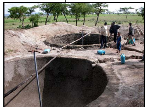
Water harvesting tanks in construction near Shashemene town in Oromiya, May 2003
